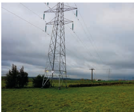
Pylons and overhead cables with 40m easement corridor cross the site
