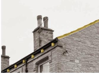
A consistent roof design with wet verge and stone dentils
