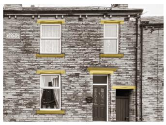
Finely finished stone lintels and sills
