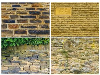
Local sandstone used for building and boundary walls, laid in a variety of bonds, with distinct variations in texture, shape and finish
