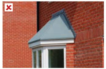
The use of poorly designed and detailed GRP elements is not acceptable.
